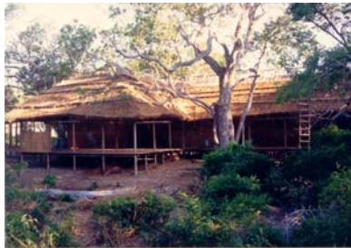
The building begins
