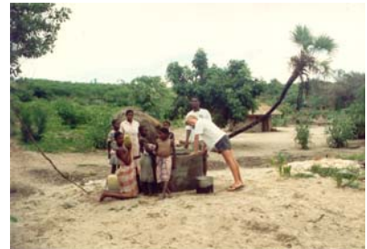
Digging a well for the villagers
