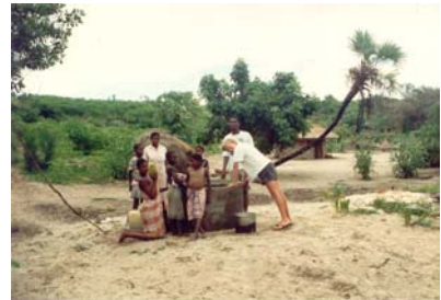
Digging a well for the villagers
